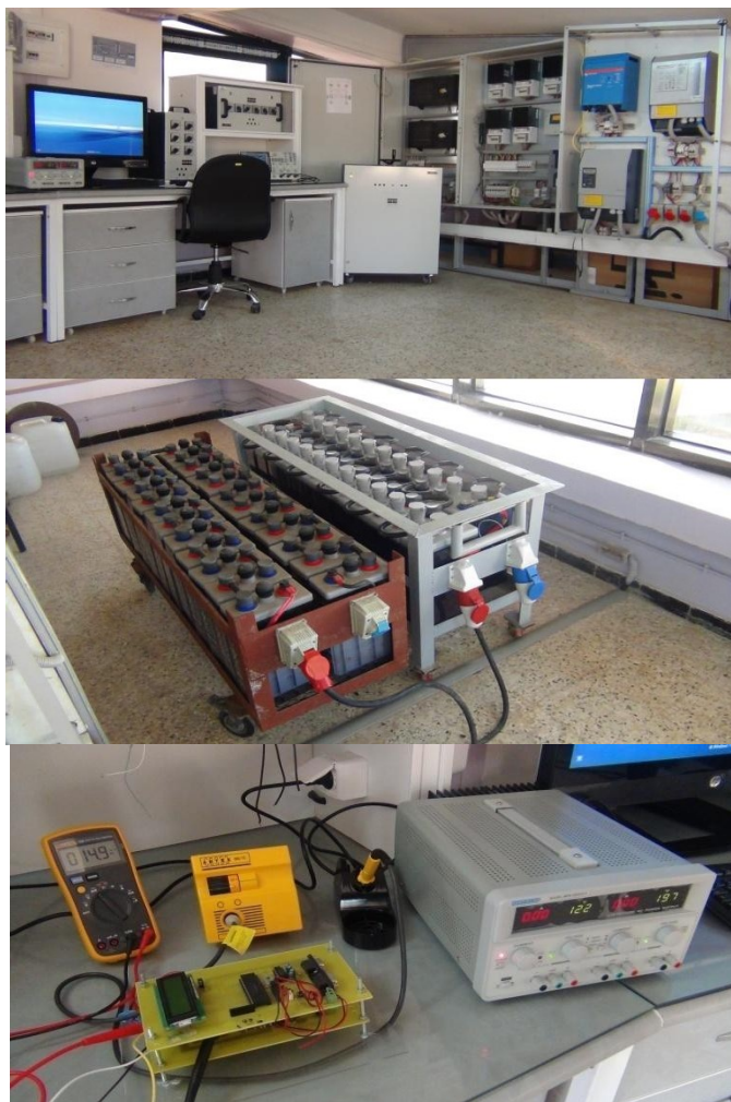
Fig.6. Photos of the PV-Wind experimental platform.
