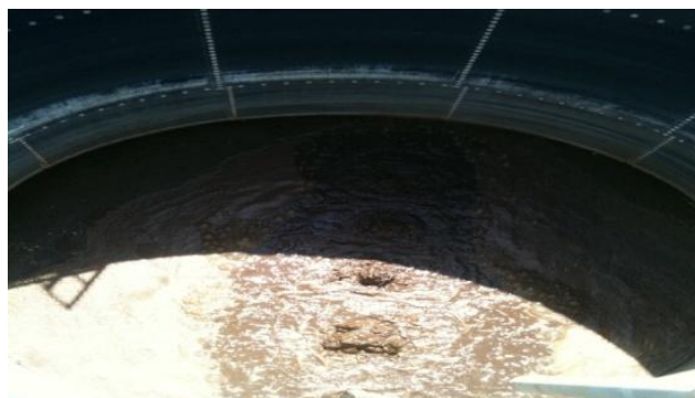
Fig.3.: Levy of sanitary water deposits
