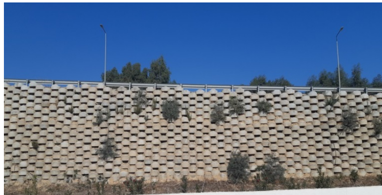
Fig.2 Development of vegetation on a RGRW on the A1 highway, Tunisia
