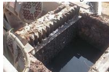
Fig.1 : photo of screen / grinder
